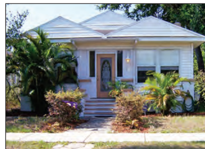
JULY: 210 13th Avenue N "Before"
