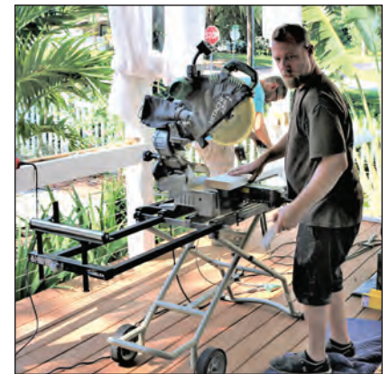
Porch carpentry underway
