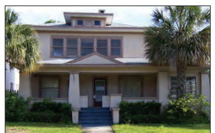
NOVEMBER: 101 10th Avenue N "Before"
