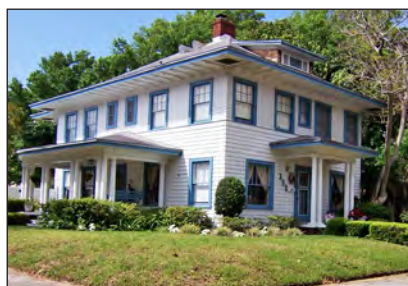
APRIL: 300 15th Street North "Before" photo
