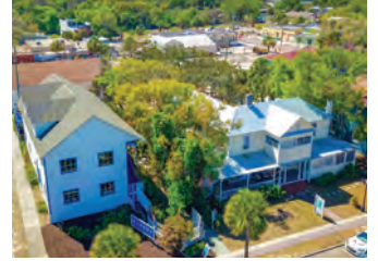
320 East Tarpon Avenue $928,000 | Web ID U7851766 Ron Goldstein 312.771.7190
