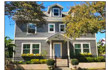
MARCH: 548 1st Street North "After" photo
