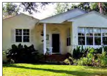
FEBRUARY: 132 24th Avenue N "Before"
