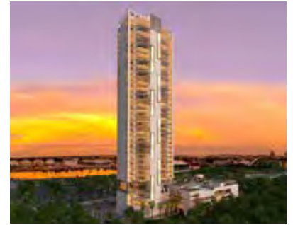
ELEVÉ 61 858 Channelside Drive - Tampa Starting in the $800s Offering 2,139 - 2,199 SF 813.510.6080 | Eleve61.com
