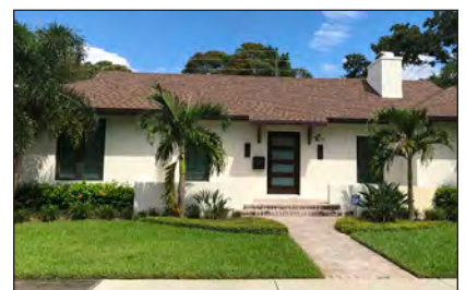
JULY: 425 21st Avenue NE "After"
