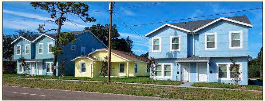
Multi-Unit Duplex on major street
