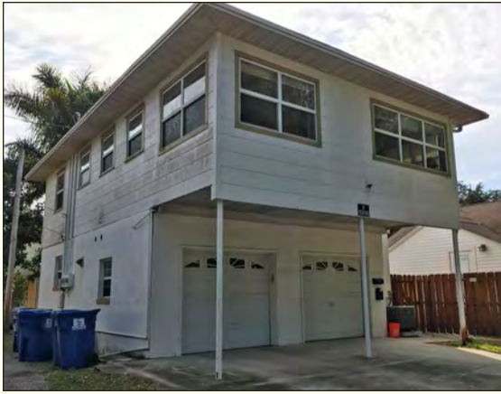
Accessory Dwelling Units (ADUs) are now largely limited to Traditional Neighborhoods, most of which have alleys. Many ADUs are garage apartments which are rented.
