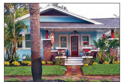
APRIL: 555 12th Avenue NE "After"
