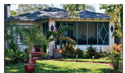
APRIL: 101 26th Avenue NE "After"
