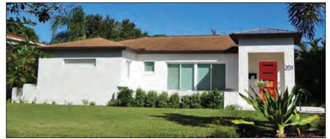
201 17th Avenue North "After" photo
