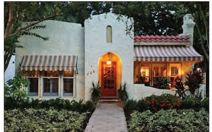
226 17th Avenue NE "After" photo
