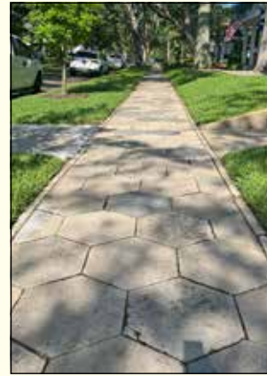
A stretch of well maintained pavers on 17th Ave NE
