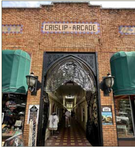
Crislip Arcade in the historic downtown strip of Central Avenue
