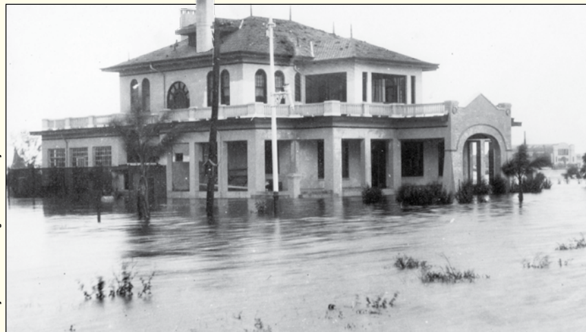
Flooding at the St. Petersburg Yacht Club after the 1921 hurricane. The club plans to raise $40 million to replace the current building to meet current FEMA and city standards.
