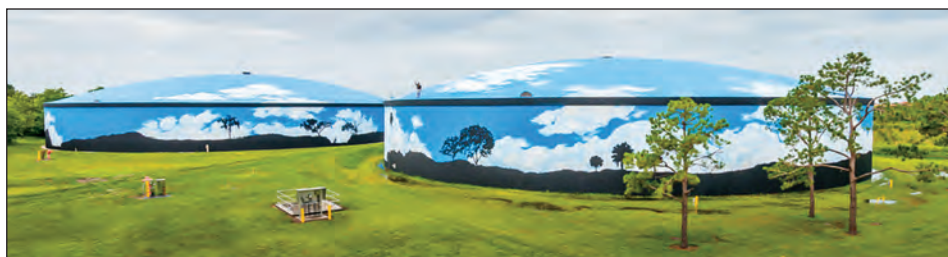
Tom Stovall stands on top of the water treatment tanks that he painted.
