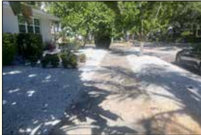
Rocks and shells can cause additional runoff and are considered impermeable according to city code.
