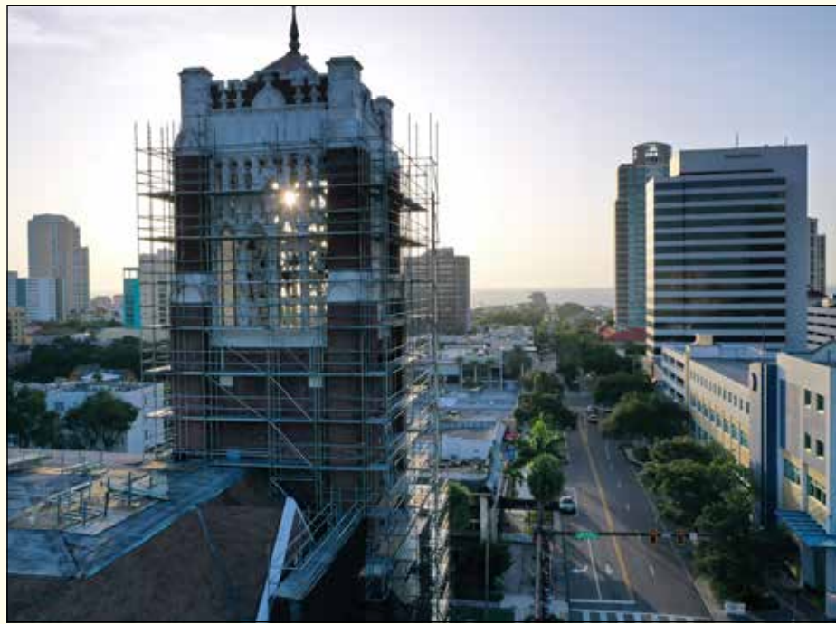
Massive scaffolding surrounds First United Methodist Church with preservation work underway.
