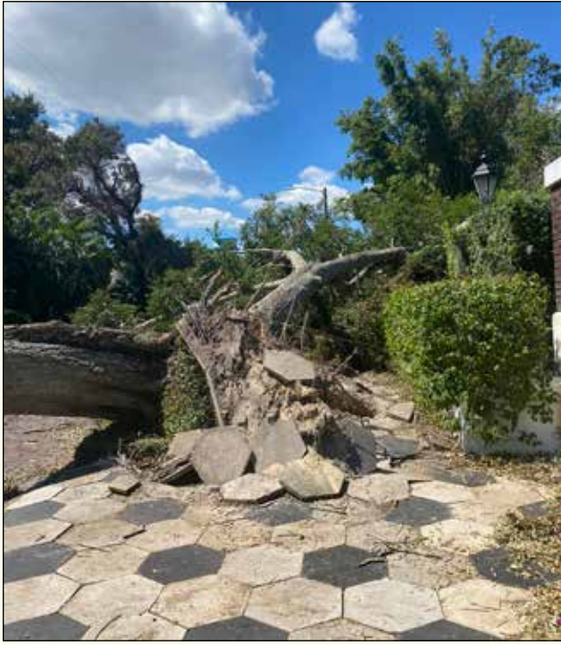
Iconic pavers disheveled by a downed tree
