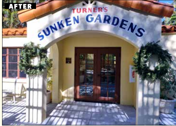
Original 1940's Turner's lettering was uncovered in renovation, now the History Center entrance.
