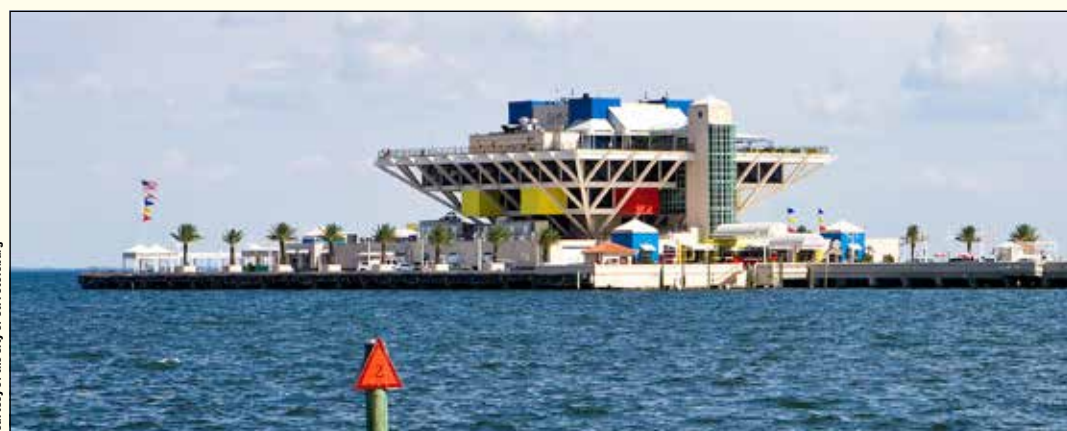
The Inverted Pyramid Pier
