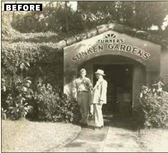
The original 1940 entrance in an historic photo
